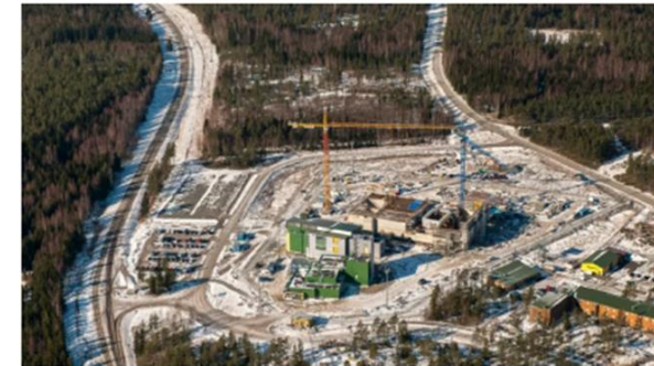
An aerial view of Onkalo, the world's first permanent depository for nuclear fuel waste, during construction. It opens later this year on the Finnish island of Olkiluoto. Tapani Karjanlahti/TVO
